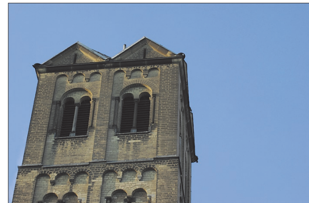
Before: The tower appears to be “falling away.”
