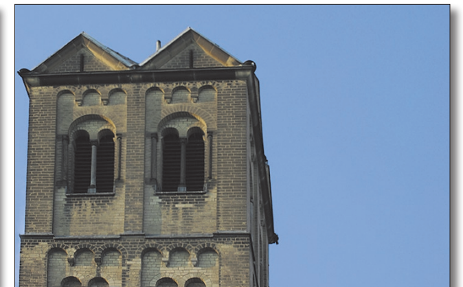
After: The same photo after repairing the perspective distortion (known as keystoneing).
